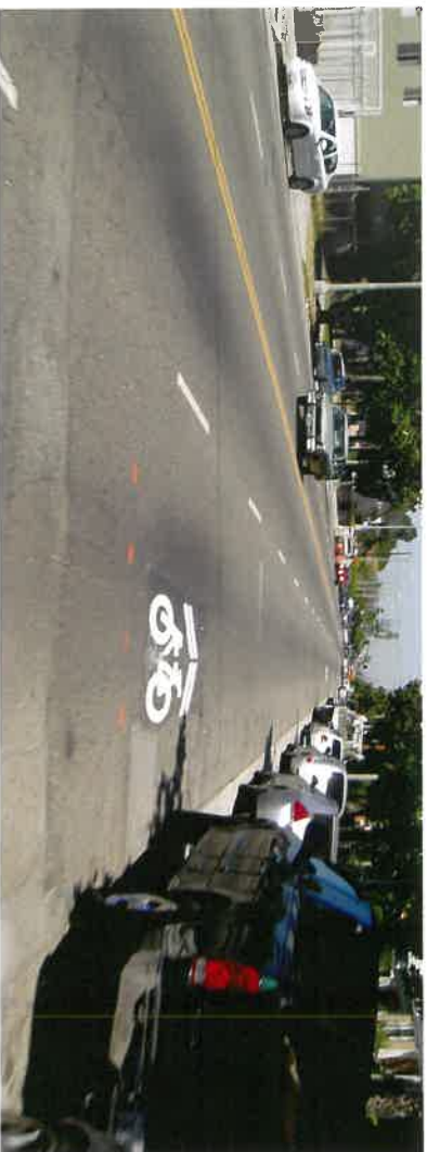
Figure 4 Adams Blvd SLM installation with orange markings to help guide video analysis measurements
